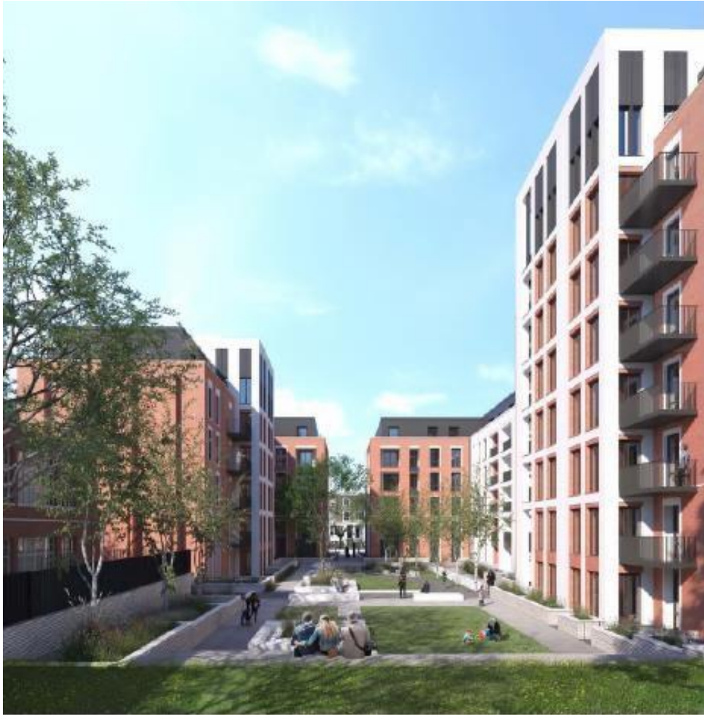
Image: View looking north into one internal courtyards between Blocks 02 and 03
